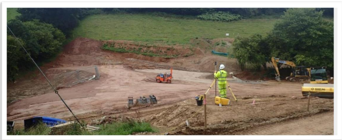
Looking east in Area 2 with the main bund taking shape.
