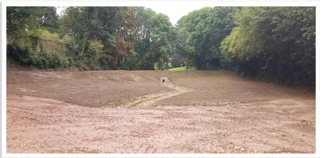
Looking south towards the substantially completed Area 1 lower bund. Grass seeding, flow control and grill to be fitted.
