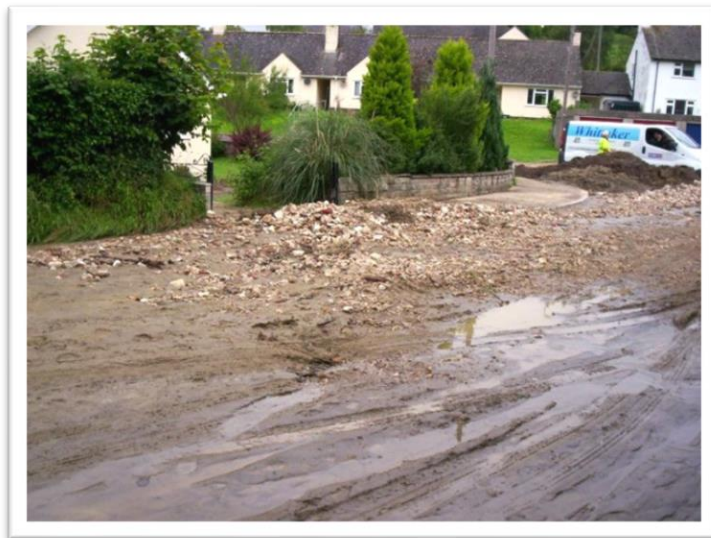
Debris that will be captured by new silt traps
