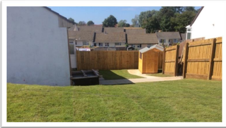
Reinstatement after completion of works
