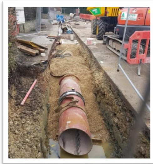
Works in progress
