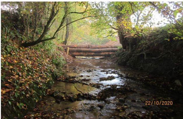
NFM interventions- New leaky dams installed on areas where high flows will be stored and slowed.
