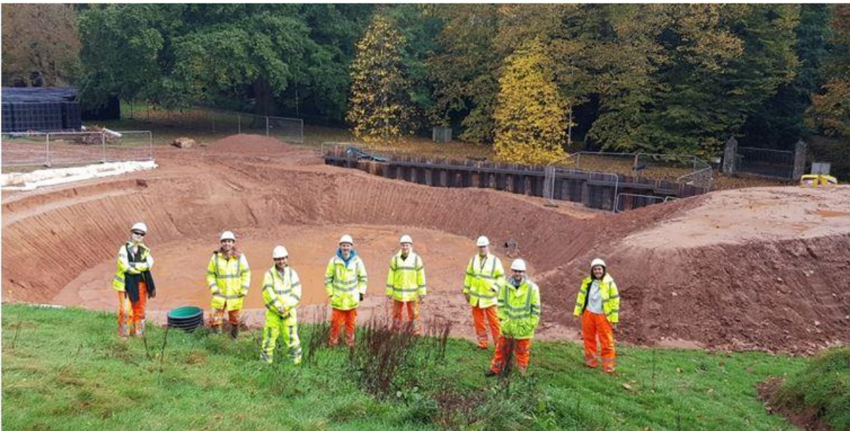
Amphitheatre storage area- Flood and Coastal Risk Management team visit
