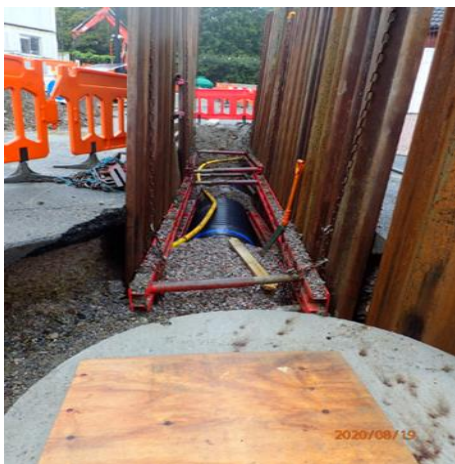
New 750mm dia. storm culvert.
