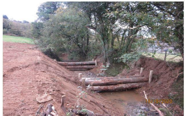
NFM interventions- New leaky dams installed on areas where high flows will be stored and slowed.
