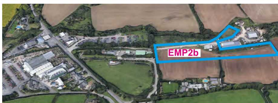
Proposed site for the extension of Dodovens Farm existing employment area
