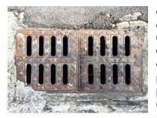
Ask your Parish Council if they employ a lengths man? A lengths man would walk the lanes checking that the drains and buddles are free from leaf and other obstructions to allow the free run of rain water into the drains. What is a buddle? "Buddle holes are holes or pipes that carry water through a hedge or a bank as part of road drainage." The lengths man must be **Chapter 8** trained (Chapter 8 refers to the Traffic Safety Measures and Signs for Road Works and
